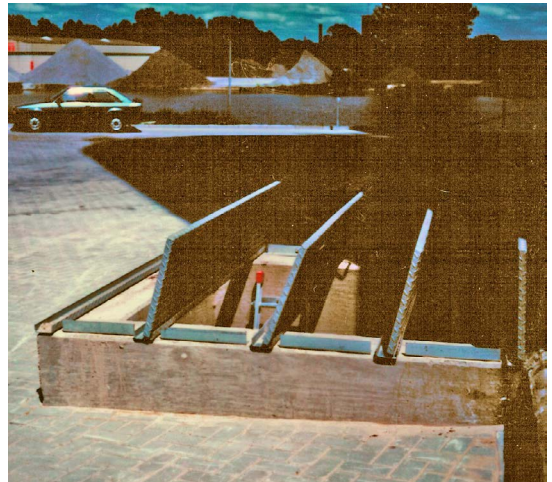
Figure 38: Emergency exit from a silo cellar, which also serves as pressure venting. (Prof. Siegfried Radandt)
