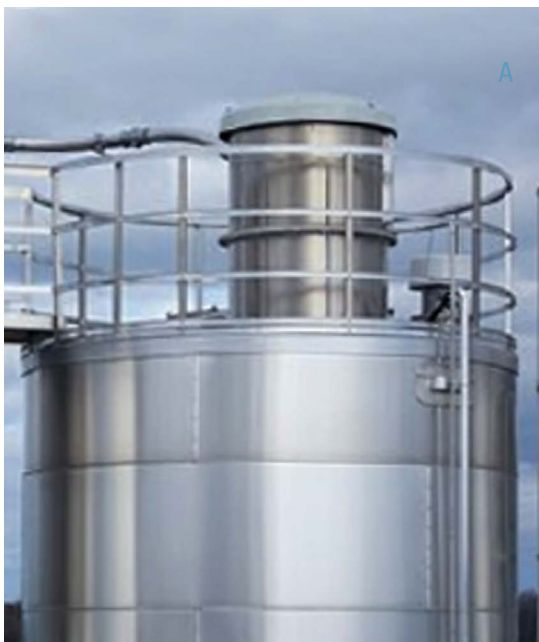
Figure 15: Silo ventilation filters designed as purge air filters (A, B: bag filter, C: pocket filter) (A, B: AZO GmbH + Co. KG, C: WAM GmbH)
