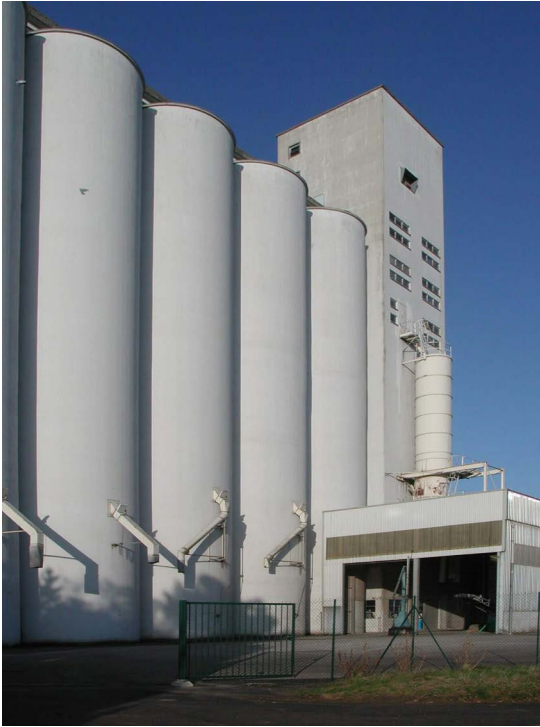
Figure 37: Silos with machine building and pressure relief areas (Prof. Siegfried Radandt)
