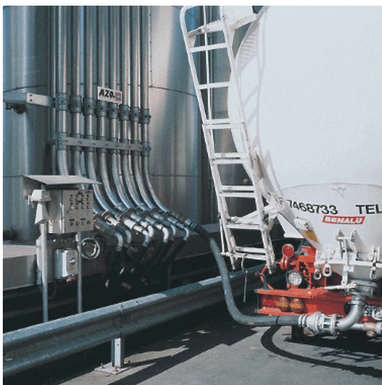
Figure 12: Silo vehicle connected to filling lines of storage silos. (AZO GmbH + Co. KG)
