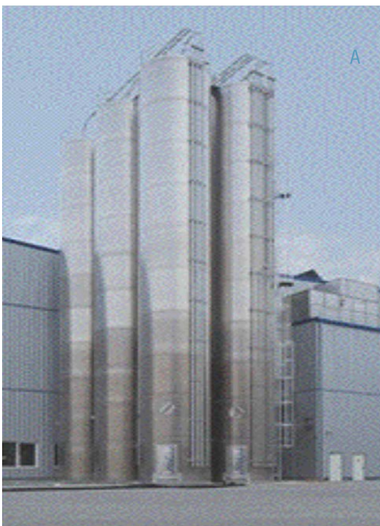
Figure 16: Closed storage containers made of different wall materials A: Outdoor silos aluminum/stainless steel B: Indoor silos stainless steel C: Indoor silos flexible (AZO GmbH + Co. KG)
