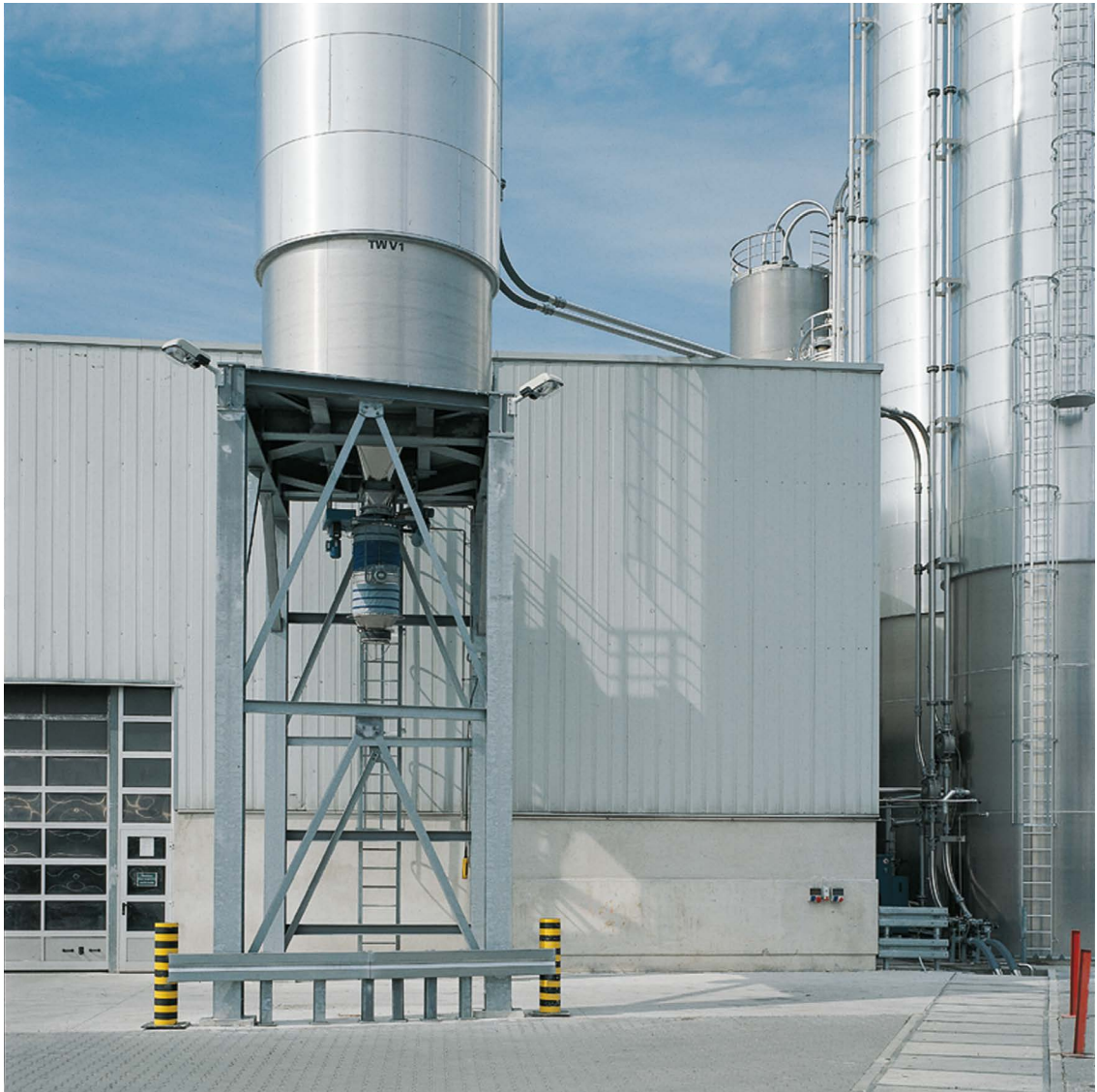
Figure 2: Storage silo with filling device for silo vehicles (AZO GmbH + Co. KG)
