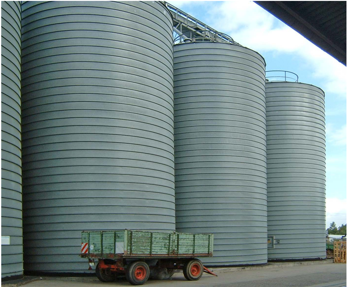
Figure 17: Flat-floor silos with integrated clearing screws (Prof. Siegfried Radandt)
