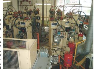
and since propane and butane are heavier than air, the lower part of the filling area up to a height of 1 m over the highest possible gas discharge position on the carousel is classified as Zone 1.
