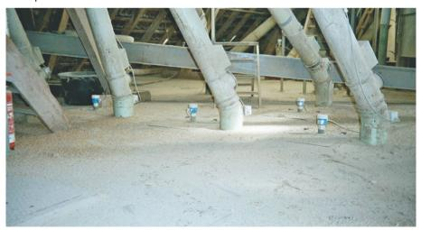
*Figure 2: Example of poor cleaning of the floor over a silo complex. Check marks are not visible anymore, therefore Zone 22*
