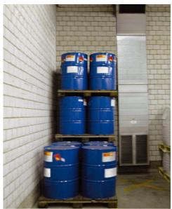
In addition an effective ventilation system has been installed and therefore the storage area is classified as nonhazardous i.e. no zone. In the absence of the ventilation system the area would be classified as Zone 2.
