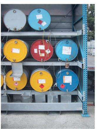
Figure 15: Flammable drum storage area with dispensing station
