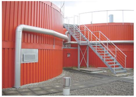
Figure 16: Two fermentation tanks with integrated gasometers<sup>1)</sup>
